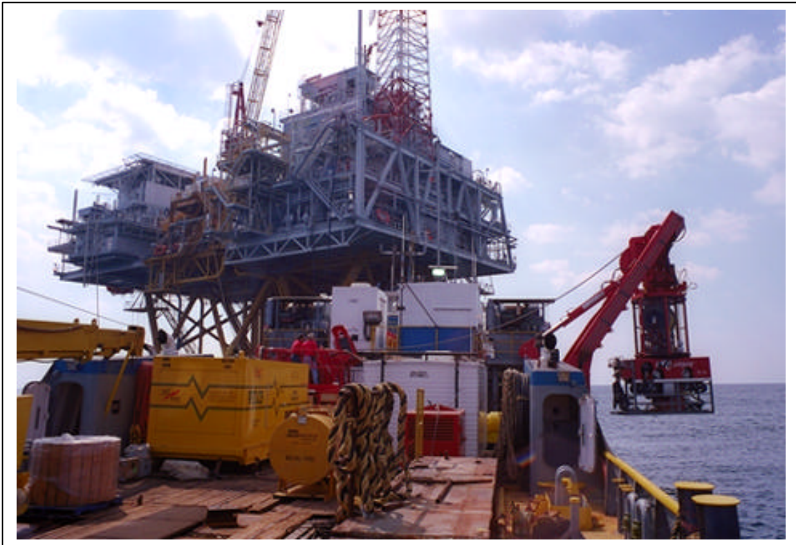
Typical offshore ROV installation
