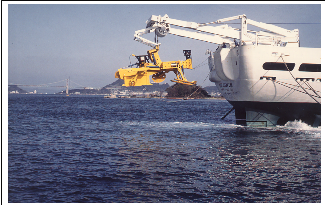
Plough and handling system aboard ship (Soil Machine Dynamics Ltd.)
